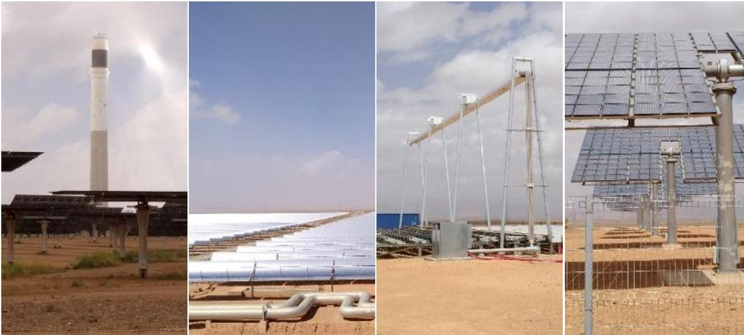
**Figure 11: Concentrating solar technologies: Solar Tower, CSP, linear Fresnel, CPV (from left to right); Ouarzazate, Morocco 2019**
